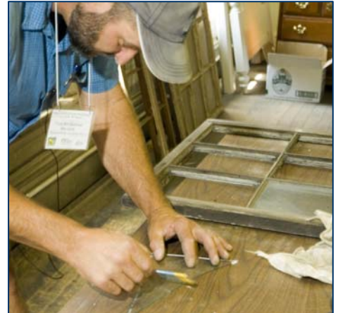
Repair of wooden windows
