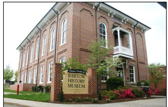
The completed 1869 courthouse will house the Bartow History Museum when open in 2011
